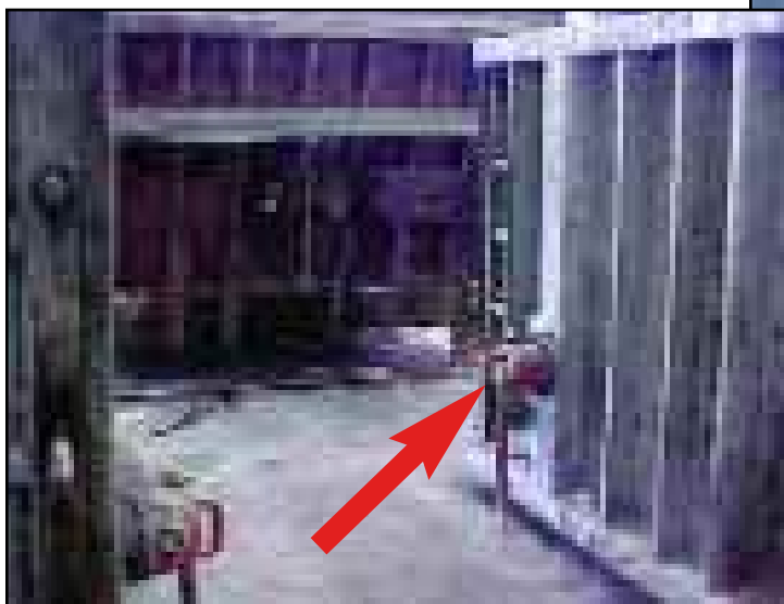
Two Model SVRLS pneumatic vibrators on lug brackets were mounted diametrically opposite on this box form.
